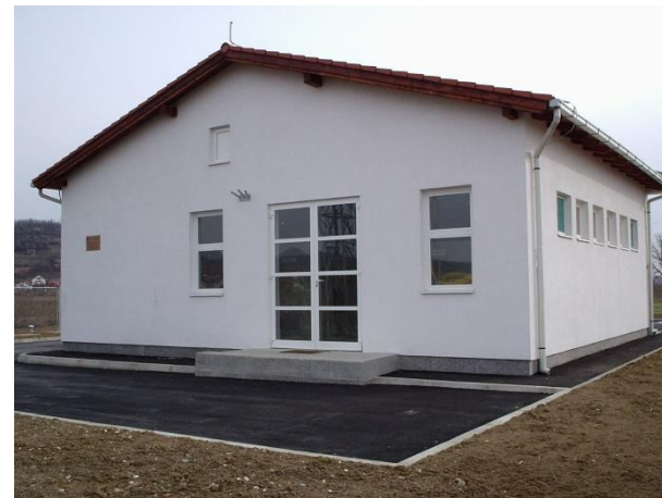
TS 35/10(20) kV SIBINJ
