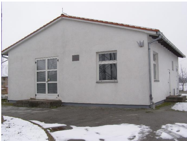
TS 35/10(20) kV TRNJANI
